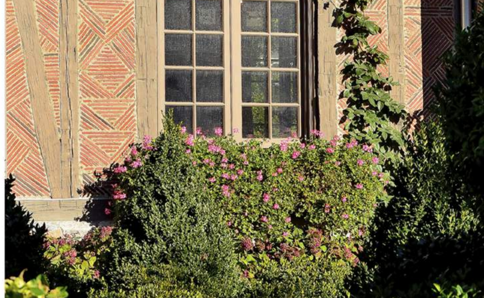
Designed by Charles Hilton Architects this project has a natural slate roof. In between the hand-hewn timbering, are Ludowici tile.
