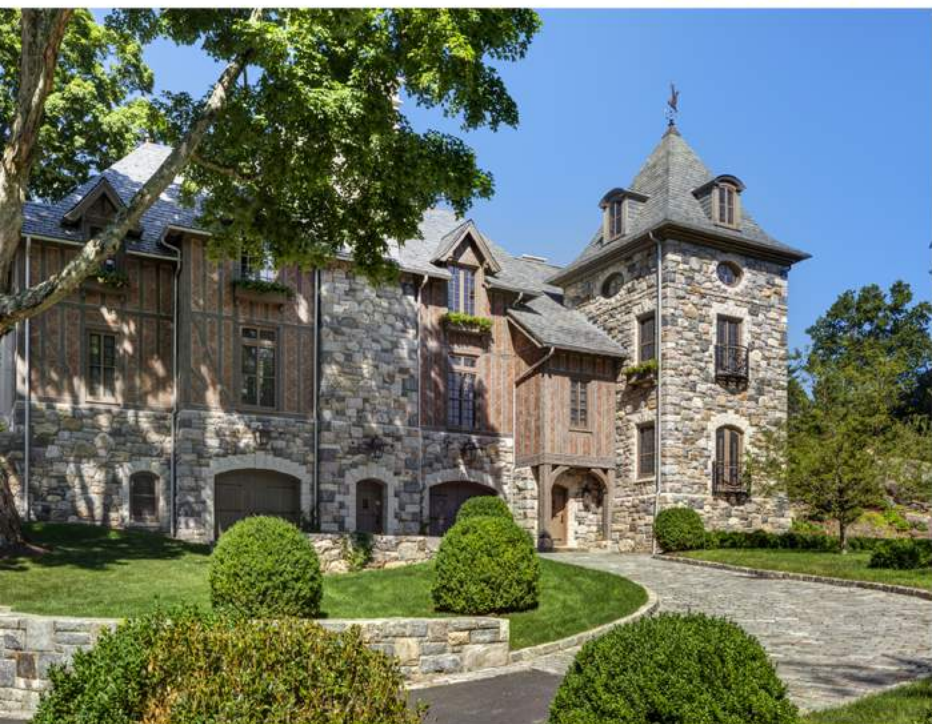
Designed by Charles Hilton Architects this project has a natural slate roof. In between the hand-hewn timbering, are Ludowici tile.
