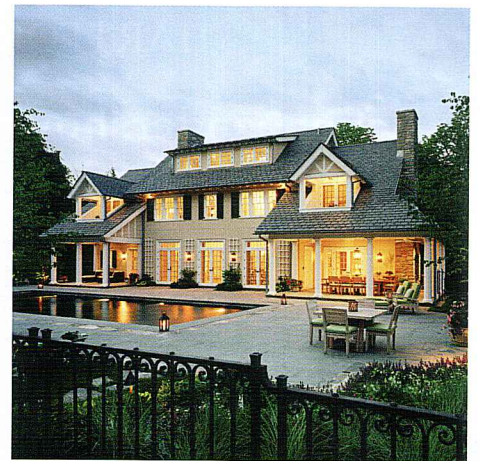
Significant rear elevation
